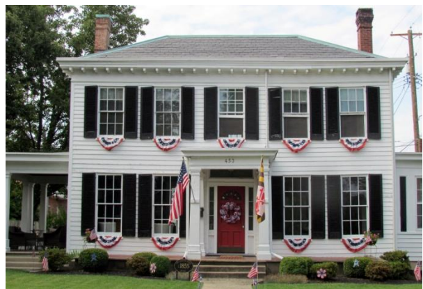
453 Congress Avenue The Carver Cobourn House, HA-543, L19, A
