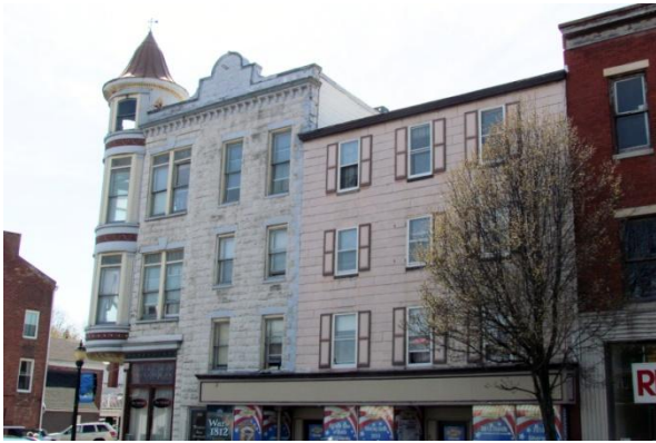
200-206 North Washington Street Maryland House Apartments, HA-1750, L47
