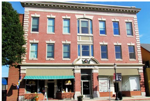
213-217 North Washington Street Masonic Temple Building, HA-1180, L49
