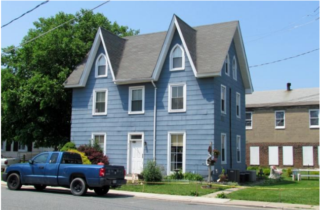
515 Franklin Street Mentzer Apartments, HA-1158
