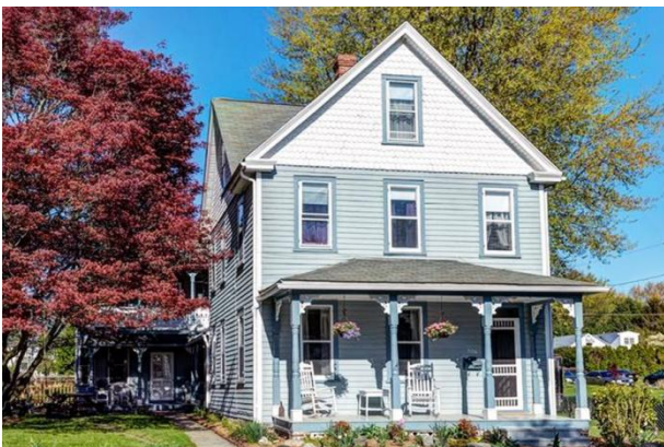
706 Market Street Brown House, HA-1176
