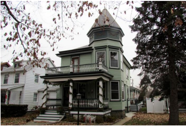
209 North Union Avenue James Fahey House, HA-1167
