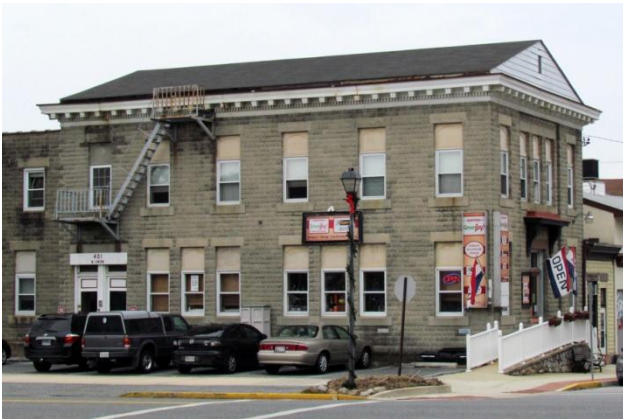
401 North Union Avenue A.P. McCombs Building, L8
