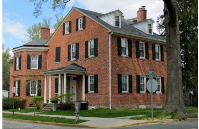
701 North Adams Street Barnes-Hopper House, HA-832, A
