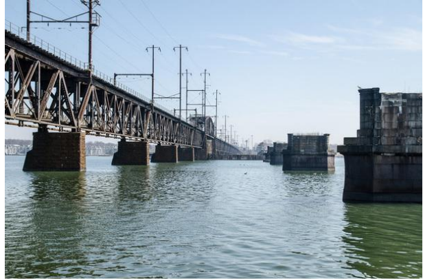
Bridge Over Susquehanna River PW&B Bridge, HA-1712, L2
