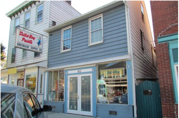
102 North Washington Street Asher's Paint Store, HA-805
