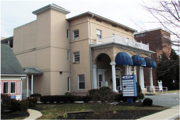
421 South Union Avenue Colonial Hotel Building, L32
