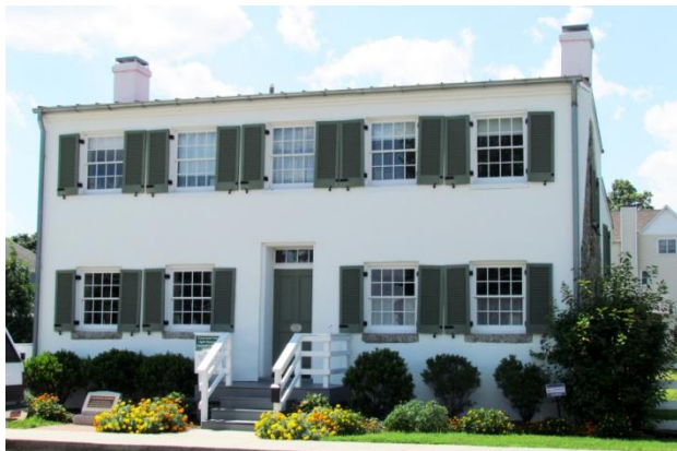
714-722 Concord Street Lighthouse Keeper's House, HA-536, L42
