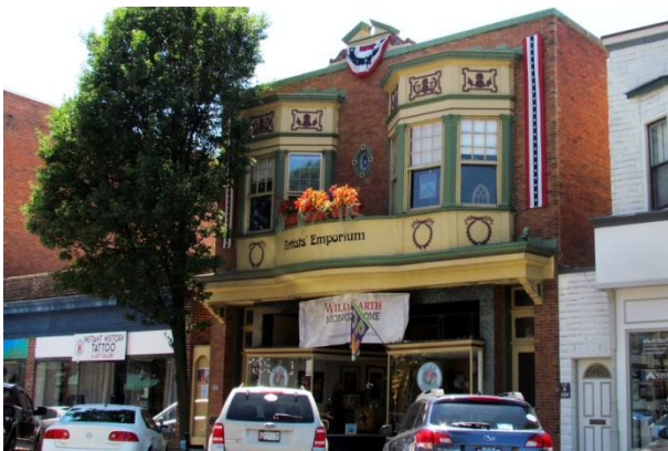
220 North Washington Street Newmeyer Building, HA-1123, L48
