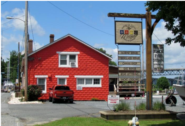
723 Water Street Abbott's Ice House, HA-1182
