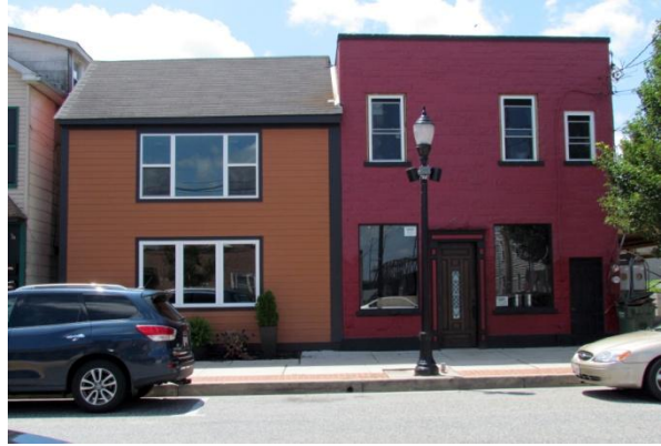
410-412 St. John Street Rodia Shop, HA-791
