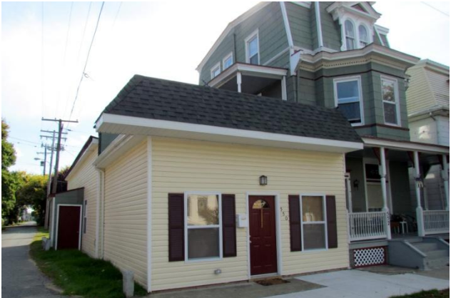
550-552 Franklin Street Joseph Good House and Store, HA-1160
