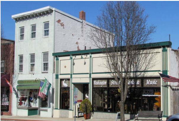
131 North Washington Street Bata Shoe Building, HA-1114
