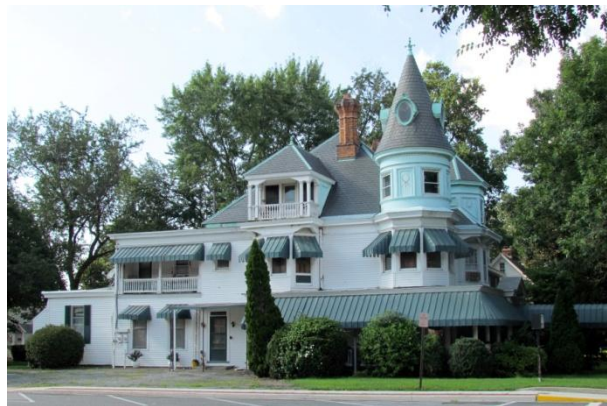
200 North Union Avenue Seneca Mansion, HA-815, L14, A
