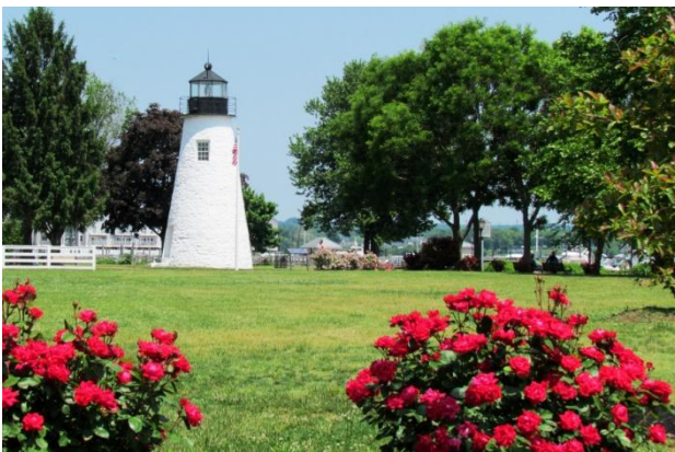
700 Concord Street Concord Point Lighthouse, HA-251, L41
