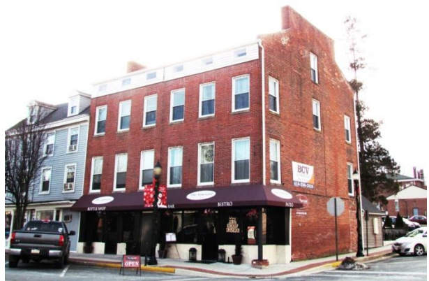
142 North Washington Street Sawyer Building, HA-801, L45, A
