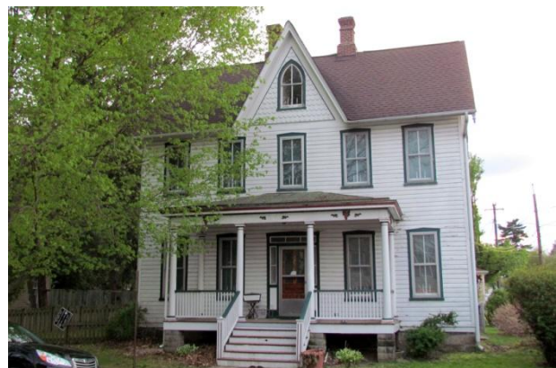
200 South Washington Street Asher House, HA-1130
