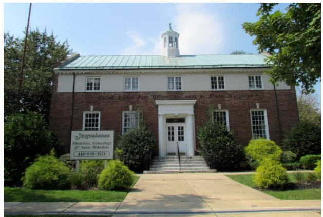
308 North Union Avenue Old Post Office Building, HA-1566, L10
