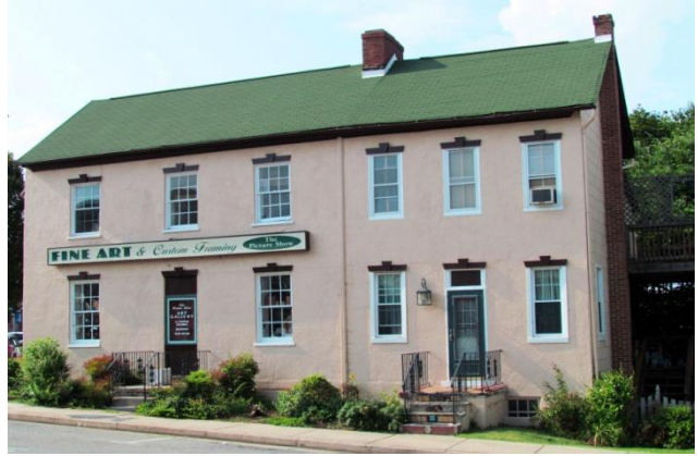
301 St. John Street Barnes-Boyd House, HA-795, L52, SW
