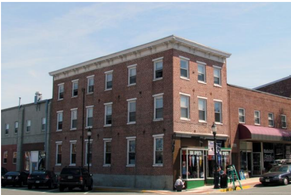
141 North Washington Street Ada Asher Building, HA-1179
