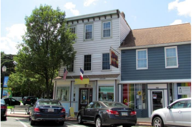
100 North Washington Street Asher Building, HA-1178
