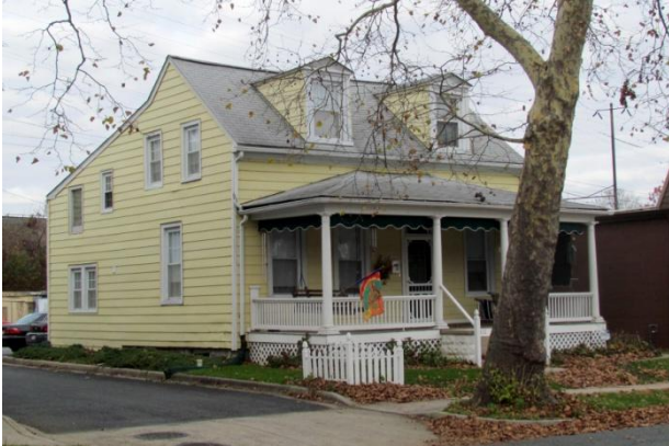
511 Warren Street Beachley House, HA-1163
